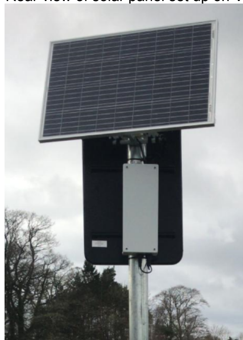
Rear view of solar panel set up on VMS
